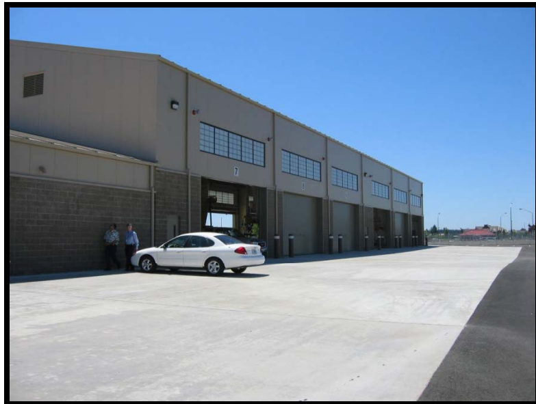
Tactical Equipment Maintenance Facility
